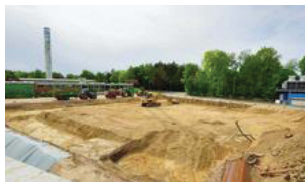
CSSB construction site on the DESY campus in May 2014 (viewed from the PETRA III tunnel).
