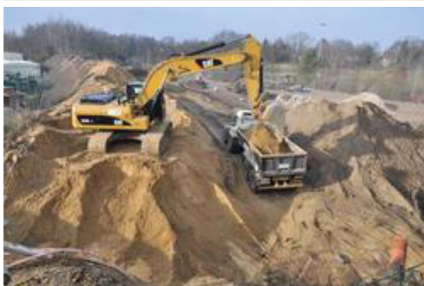
Construction site at the PXE east site (top) and north (bottom) on 7 February 2014.
