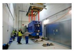
The first undulator frames have arrived at the SwissFEL building. They will take around six months to assemble, after which the finished undulators will be taken to the SwissFEL accelerator tunnel for installation.
