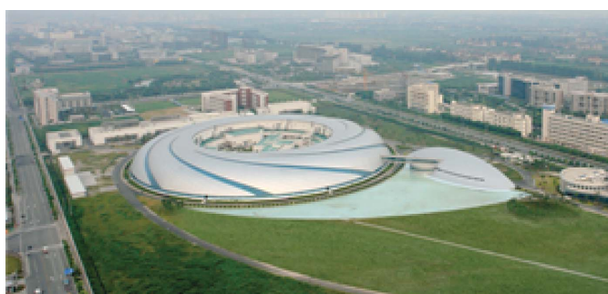
The SSRF building housing the accelerator complex.
