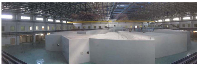
A view of the SESAME hall with completed shielding structure. The beamline apertures are clearly visible.
