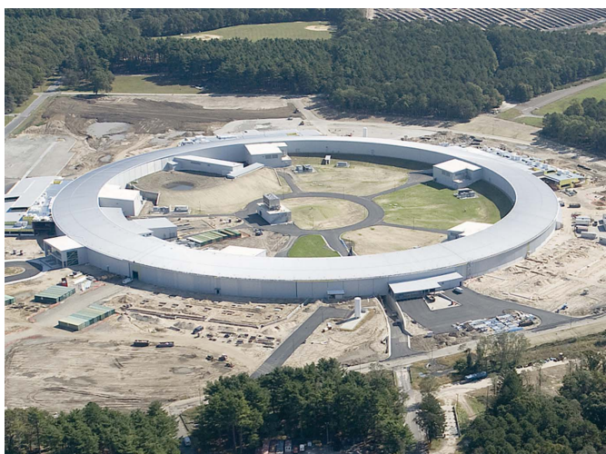
A recent aerial view of NSLS-II.
