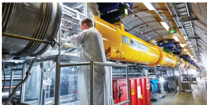
Technicians connect two accelerator modules in the European XFEL tunnel. (Courtesy of Heiner Müller-Elsner, European XFEL.)
